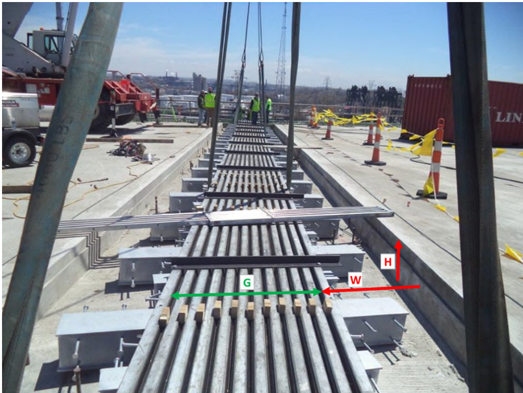
Figure 8: Joint Blockout
